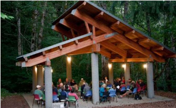
Group Shelter - Interesting Architectural Character
