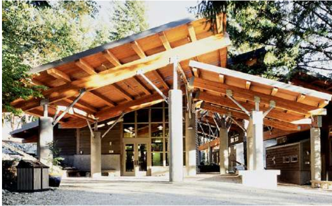
Interesting Architectural Character
