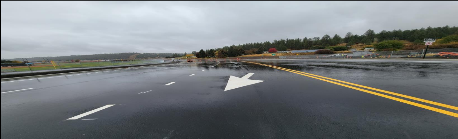
Past Project- Bigelow Gulch Project 6
