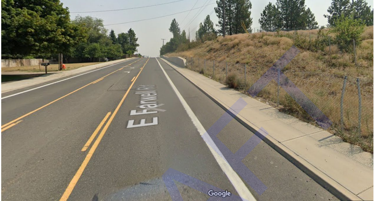
E Farwell Rd. in North Spokane County. Speed limit 35 mph
