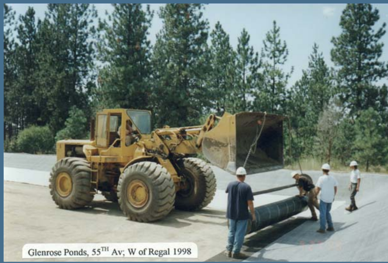
Installation of pond liner at 55 th evaporation pond.
