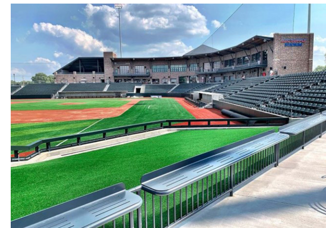
Image of Elevated 360 Degree Concourse With Drink Rail
