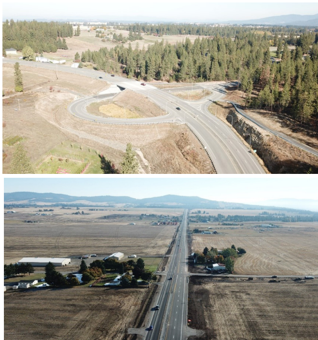
Figure 3: Completion of the grade separated intersection at Bigelow Gulch Road and Forker Road in 2019 (top) and reconstruction of a section of Bigelow Gulch Road between Argonne Road and Forker Road in 2019 (bottom)
