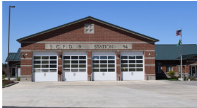
Figure 14: Spokane Valley Fire Department Station 9
