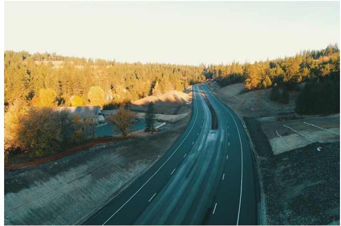
Figure 8: Improved section with wide shoulders and median
