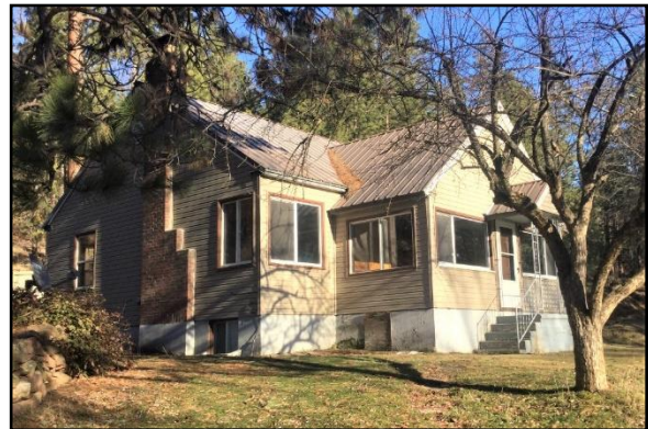
Figure 5.2-10. Residence at 2018 S Zephyr Rd., facade and northwest elevation; view east.
