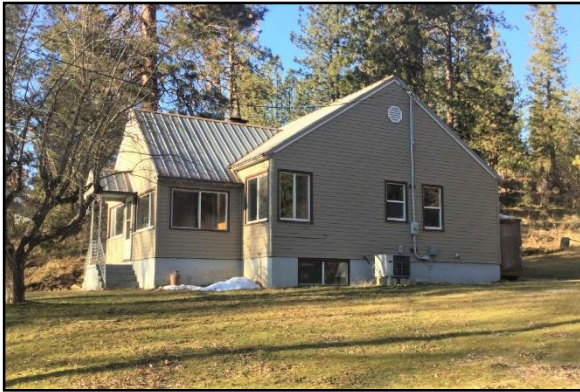
Figure 5.2-7. Residence at 2018 S Zephyr Rd., facade and southeast elevation; view north.
