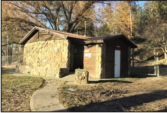
Figure 5.2-5. Restroom at 3707 S Zephyr Rd., facade and southeast elevation; view northwest.
