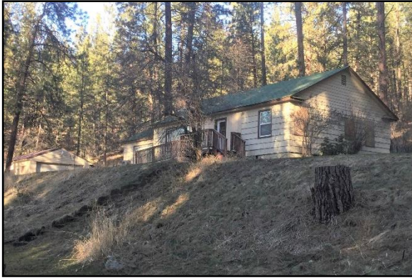
Figure 5.2-3. Residential building/office at 3707 S Zephyr Rd., facade and southeast elevation with detached garage minimally visible ( left ); view north.
