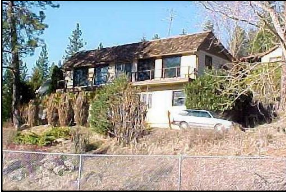
Figure 5.2-11. Residence at 2014 S Zephyr Rd., southwest and southeast elevations; view north.
