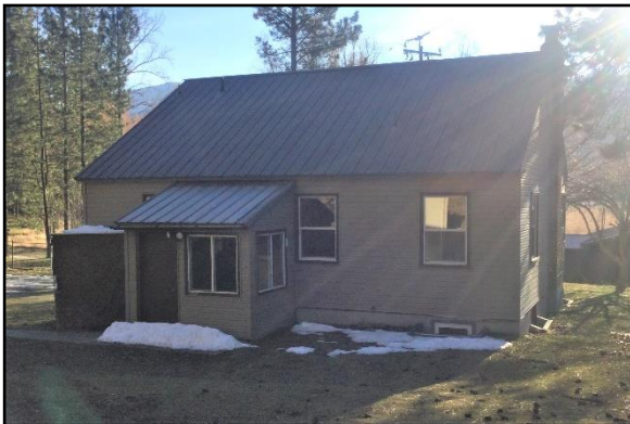
Figure 5.2-9. Residence at 2018 S Zephyr Rd., northeast and northwest elevations; view south.
