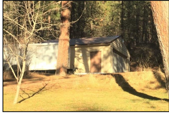
Figure 5.2-4. Garage at 3707 S Zephyr Rd., southwest and southeast elevations; view northeast.
