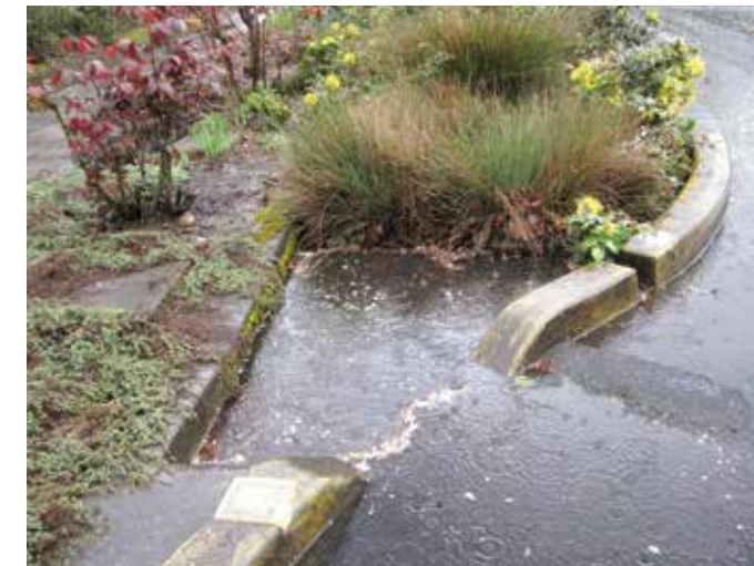
Bioretention facility in Spokane
