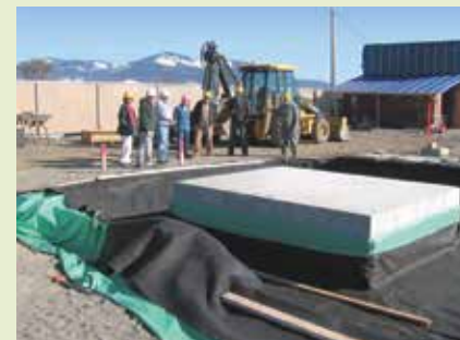
Poly-geotextile containment
