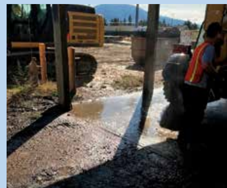
Vehicle wash water should not flow off washpad or discharge to the ground
