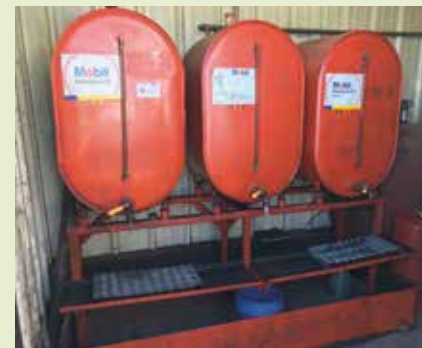
Metal containment for drums/tanks
