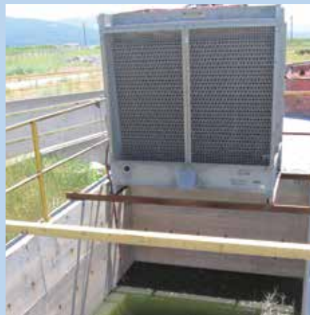
Approved wastewater retention pit with mechanical evaporator
