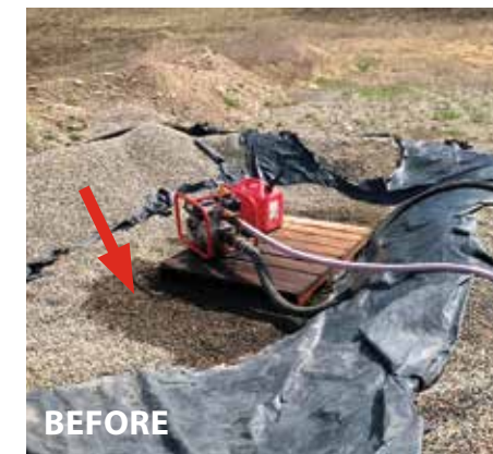
Gasoline spill before clean-up
