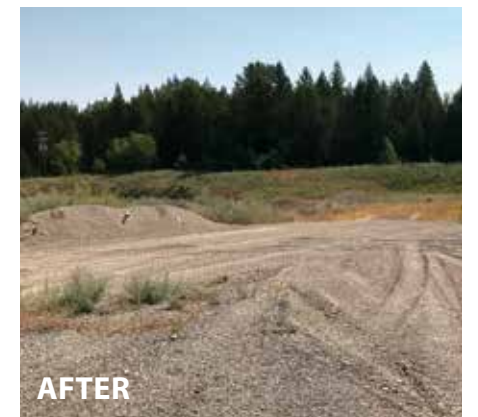
Gasoline spill cleaned up
