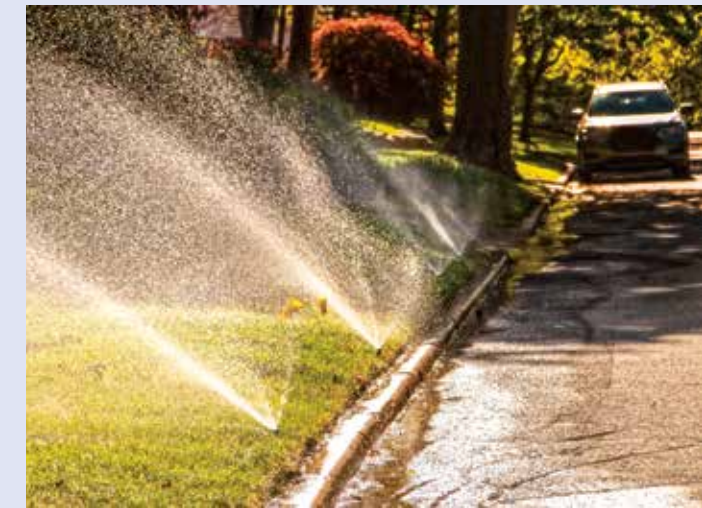
WATER WASTE Once you have efficient sprinkler heads to help reduce overwatering, pay attention to other wasteful scenarios such as overspray, misting, and runoff.
