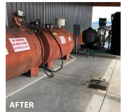
New pad, under cover, with grit chamber/blind sump
