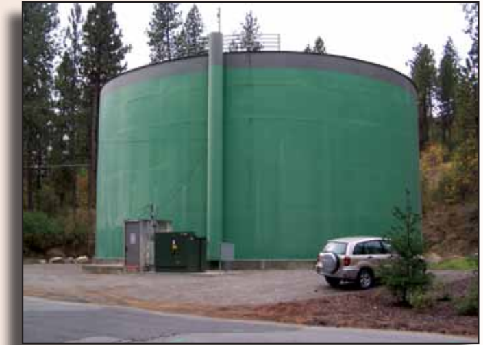
Public water purveyors pump & store Aquifer water.
