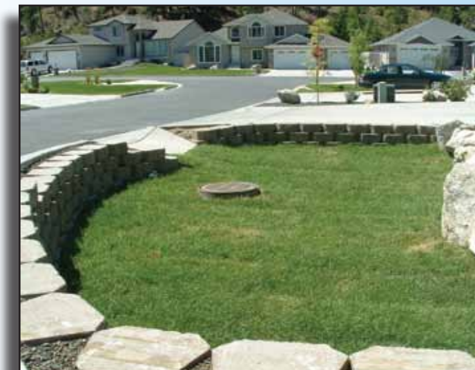
Stormwater swales and drywells recharge the Aquifer.
