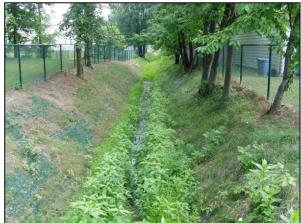
Figure 3. Ditch MS4 outfall
