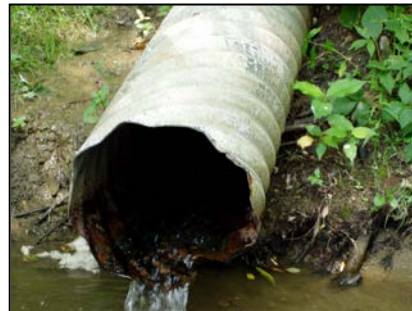
CMP (Corrugated Metal Pipe)
