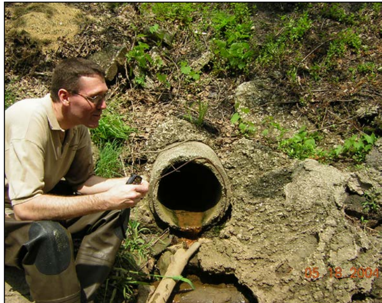
Figure 12. Dry weather field inspection
