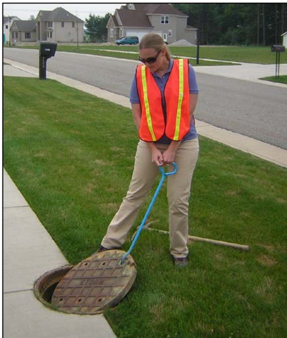
Figure 14. Removing storm drain lid
