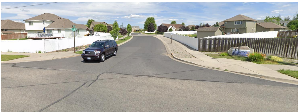
Curb ramps at the corner of 5 Mile Road and Roger Dr., rated 4 out of 5.
