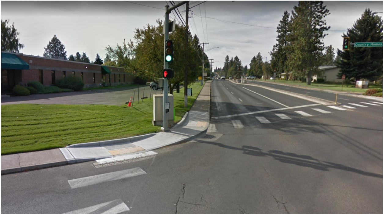
One of the 15 curb ramp improvements at signalized intersections from the 2017 Spokane County Signal Safety Project.
